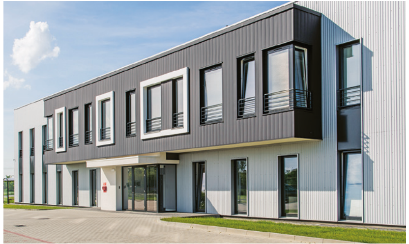
Beckers Poland: Beckry®Tex C topcoat on cladding painted at ArcelorMittal Poland
