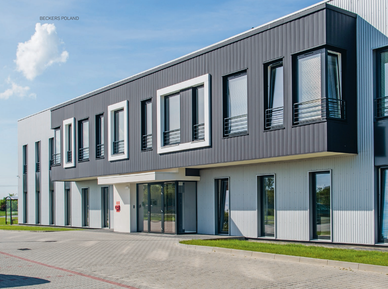
The cladding is painted in the Beckry®Tex system, coated at ArcelorMittal Poland and profiled at Blachy Pruszyński.
