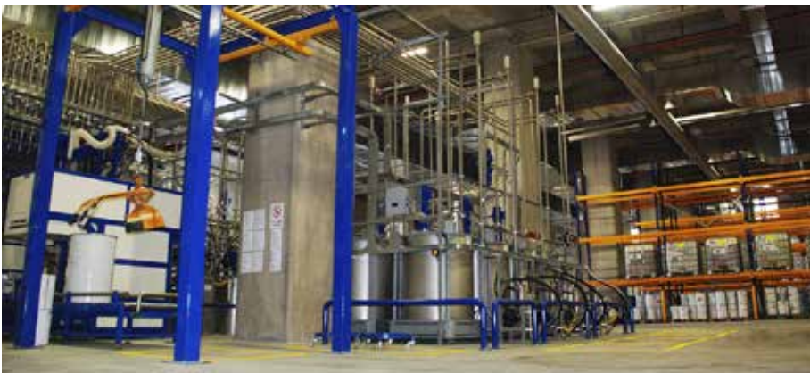
The Beckry® Mix unit at Beckers Turkey.
