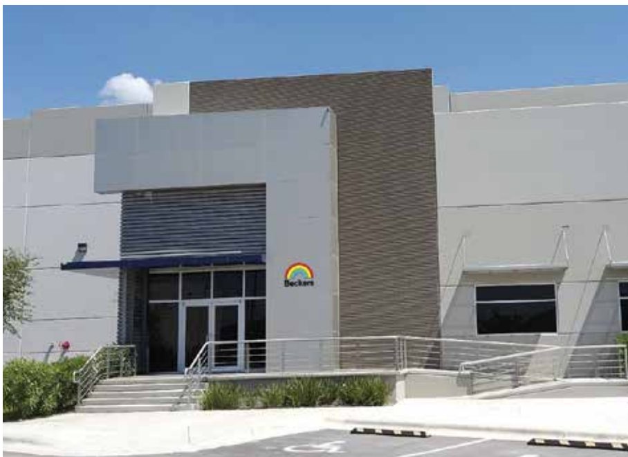
Beckers' new site in Monterrey, Mexico.
